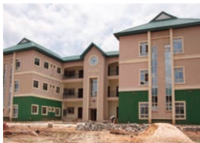
Anambra State University teaching hospital in Awka, which is nearing completion
