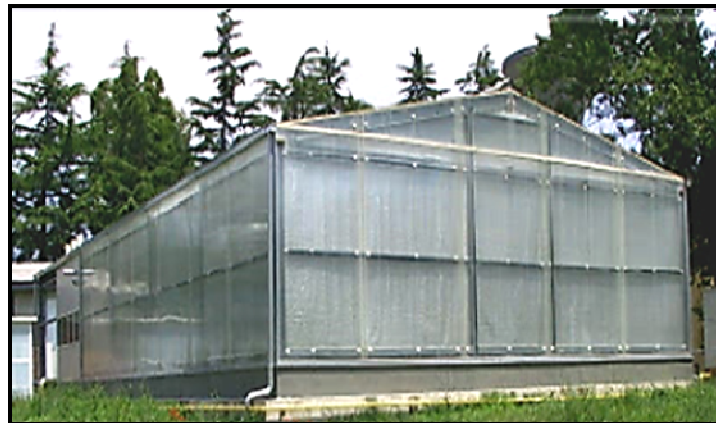
Figure R2: Containment greenhouse (P 2 level) at ENEA Casaccia Research Center, Rome.
