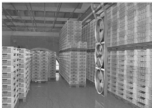
Figure 3.15 New technology for air ventilation in a grapes dehydration facility. (For a colour version of this figure, please see the colour plate section.)
