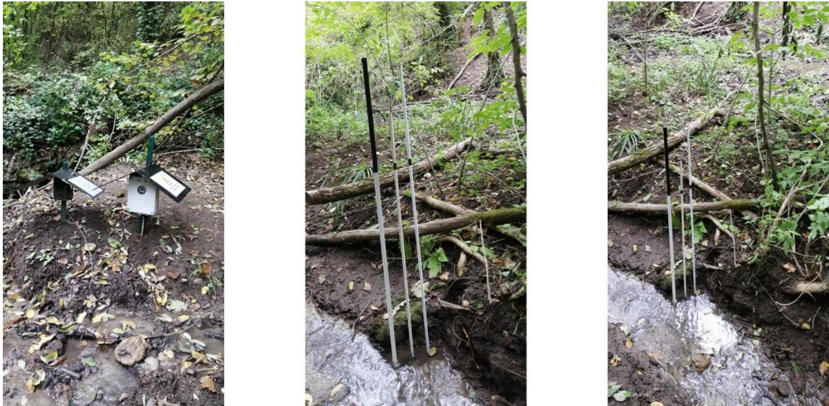
Figure 4.1. An example of stage-cam system installed at the Montecalvello basin.
