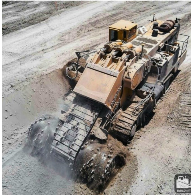
Figure 2.10. Self-moving industrial trencher.
