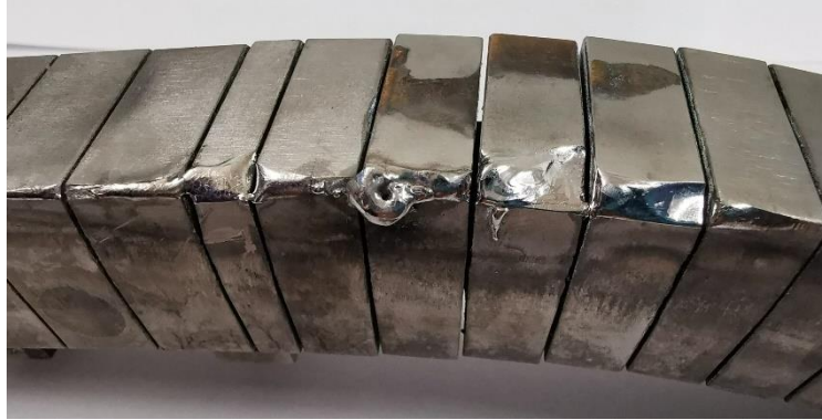
Figure 1.3 Damage of EAST target plate material caused by the plasma heat flux
