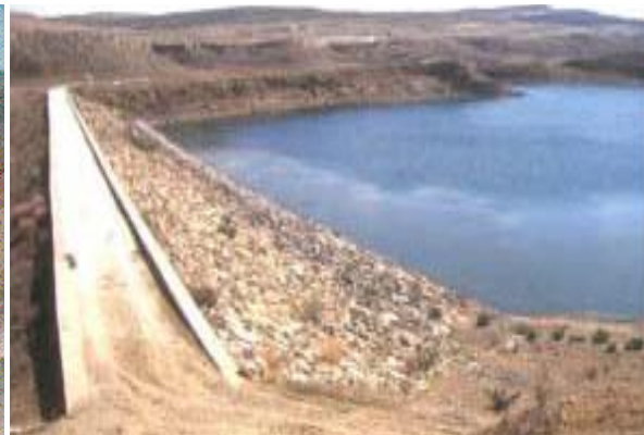
Photo 3.3 El Morra reservoir
