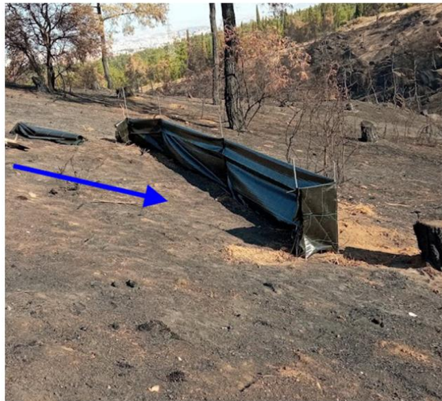
Figure 1.3: Silt fence method. Source: Kastridis et al. 2022.
