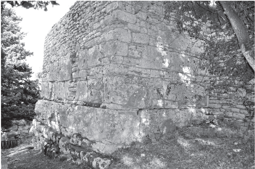
Figure 16.5. Tower 2. First phase of the city wall (© S. De Vincenzo).
