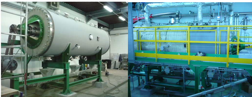
Fig.20 SSF prototypal 9m 3 bioreactor during construction (left) and refining by insulation covering of the vessel (right).
