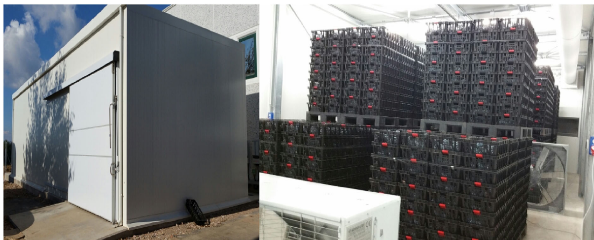
Figure 1. External and internal views of the new commercial fruttaia where the air distribution was studied. In the right-hand picture, the white perforated air duct hanging from the ceiling is shown.
