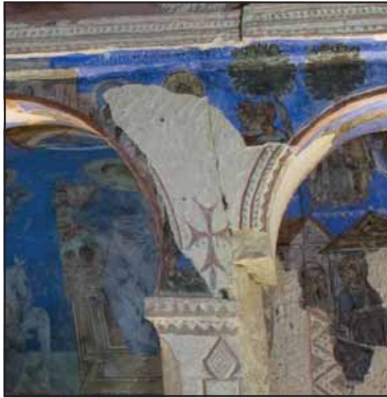
Fig. 8 Göreme Open Air Museum, New Church of Tokalı. The cracks on the rocky support in the second arch above the lacuna of the pillar.
