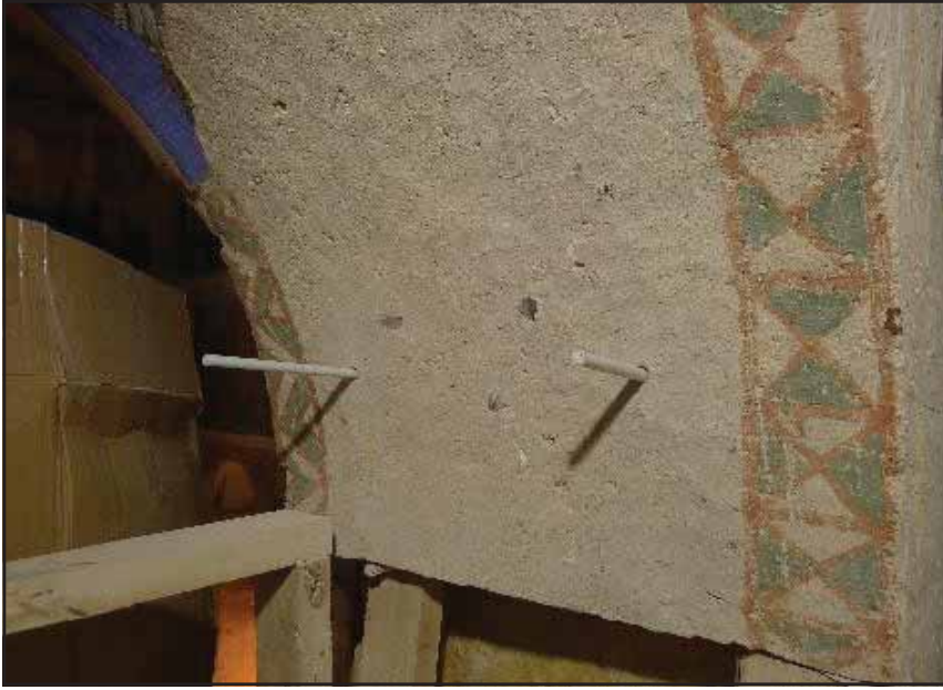
Fig. 9: Göreme Open Air Museum, New Church of Tokalı. Secon pillar, intervention with the insertion of 2 dowel rods.
