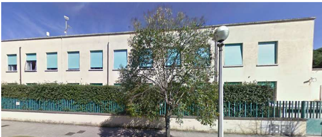
Figure 30: View of the building F from Via Vittorio Emanuele II [Google Maps].
