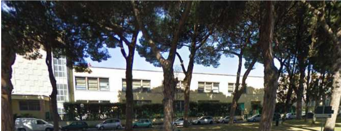
Figure 31: View of the building E from Via dei Forestali [Google Maps].
