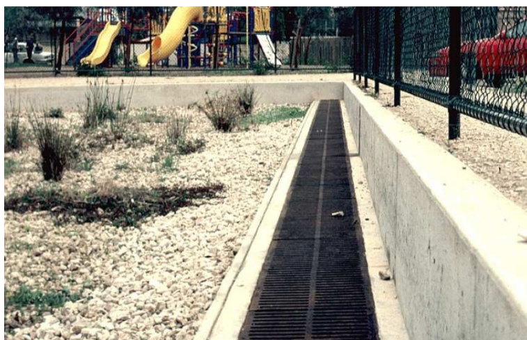
Figura 46 | infiltration measures (Tasmania, 2012)
