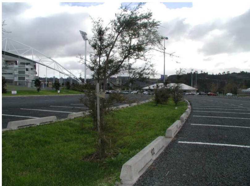
Figura 40 | bioretention swales (Tasmania, 2012)
