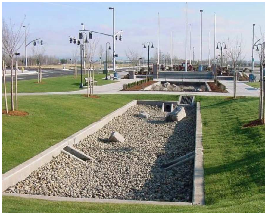
Figura 42| sand filters (Tasmania, 2012)
