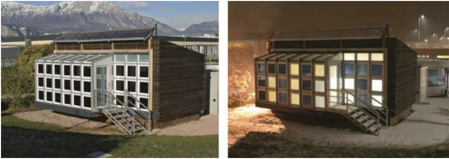
Fig. 21. Left: day view of the Dynamic Façade with all the electrochromic windows tinted. Right: night view of the Dynamic Façade with the pattern “MIT” formed by the windows.
