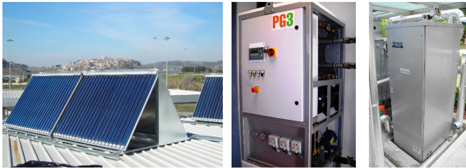
Figure 1 - (a) the solar collector; (b) the ORC unit; (c) the absorption chiller
