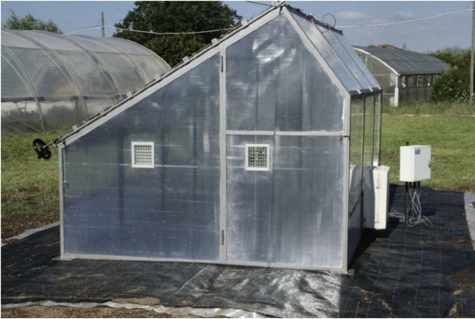
Fig. 4. Iron and glass prototype of the dynamic photovoltaic greenhouse.
